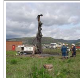
Eden Energy's rig on site in South Wales
